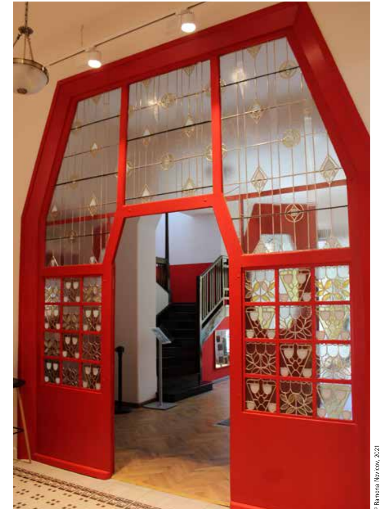
The stained-glass window in the ground-floor hallway has been accurately restored El vitrall del vestíbul de la planta baixa ha estat restaurat amb cura
