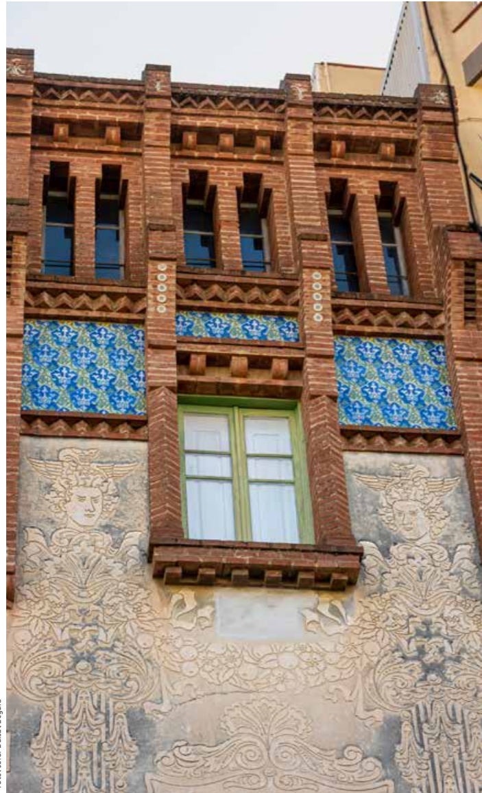
The combination of brickwork, glazed tiles and a Baroque sgraffito, lend Can Floris's façade an original look
