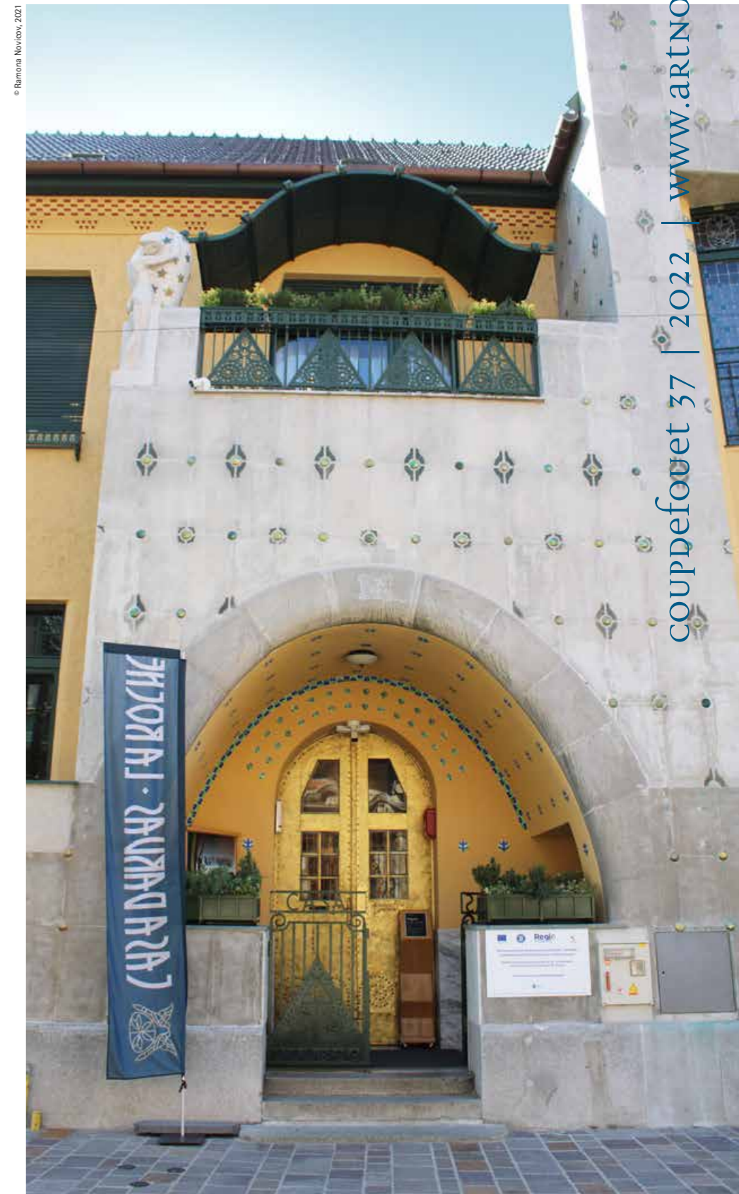
The main entrance to the museum consists of a spectacular archway and massive, brass-plated wooden door
