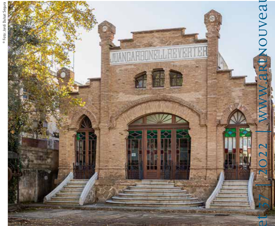
Central building of the Carbonell factory. One of the finest examples of the town's industrial Modernisme, it was designed by Josep Puig i Cadafalch in 1899
