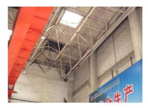
Fig. 3-3: Lower chord bending
