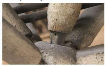
Fig. 3-8: Bolt sleeve pin is missing
