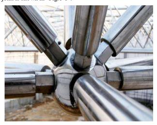
Fig. 1-1: The bolt-ball node joint
