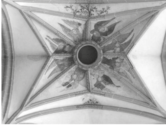
Fig. 434: Himmelloch – opening in the vault of the Holy Spirit Church in Heidelberg
