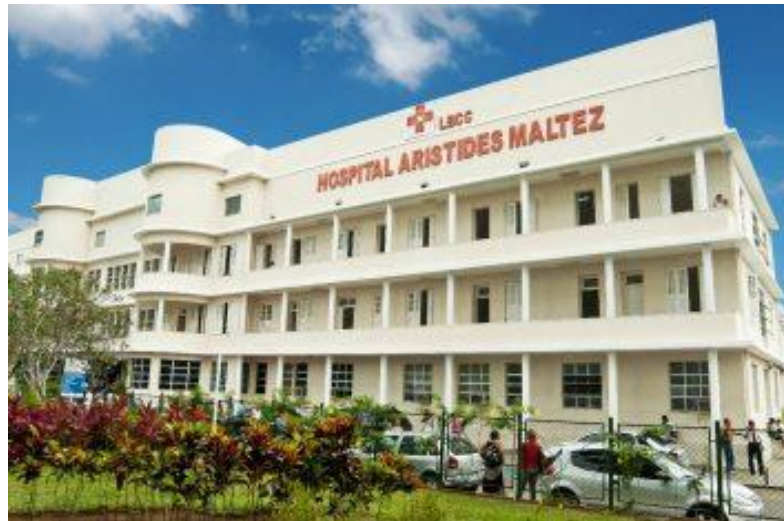
Figura 3 – Hospital Aristides Maltez
