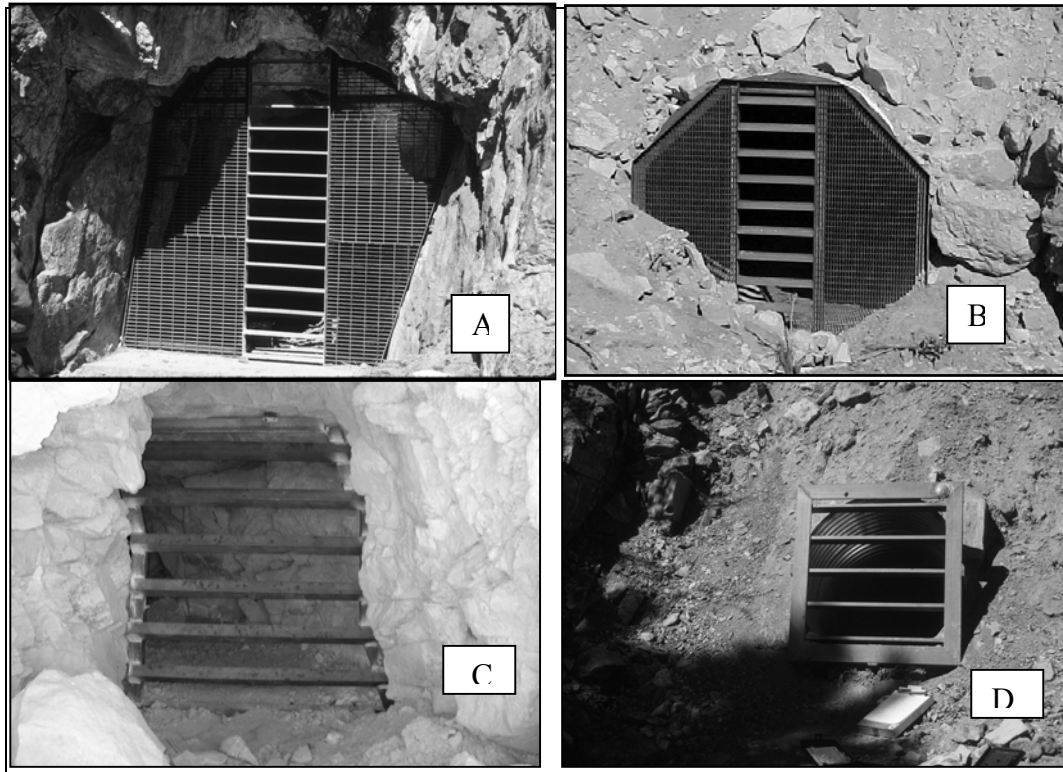
Figure 1. Styles of gate used at mines in Colorado. A) ladder, B) culvert with ladder, C) full, and D) culvert with full.
